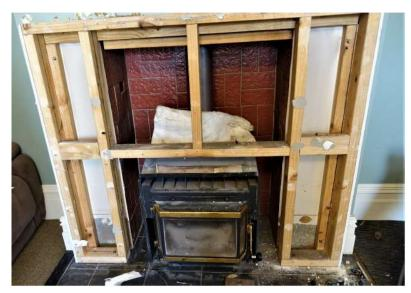
Figure 1: Photograph of the as-built woodburner
