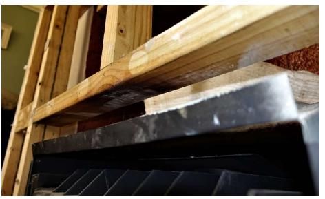
Figure 3: Photograph of a scorch mark on the timber framing
