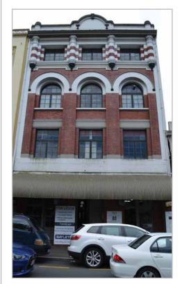
Figure 10: Works to strengthen the former Cadbury's Building at 60 Ghuznee Street, Wellington (left) are due to start in 2017. These will include strengthening the street facade with internal reinforced concrete columns and steel cross bracing, and the installation of concealed stainless steel fixings to the decorative columns at ground and third floor. The parapet will be restrained by a steel frame that will be fixed back to the existing steel and concrete structure.
