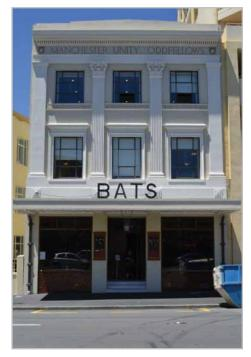
Figure 9: Bats Theatre at 1 Kent Terrace, Wellington (left) was strengthened in 2012 with new internal reinforced concrete columns and shear walls. There are new internal columns at the front elevation that continue from ground to roof level and support the parapet and facade. These have been designed so that they do not alter the street facade of the building.
